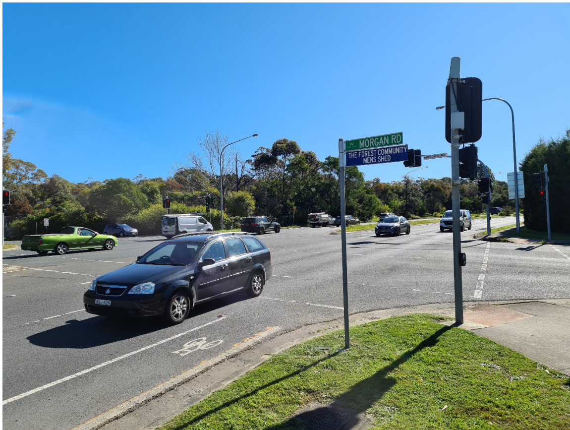
Figure 12 Existing pedestrian and cyclist facilities
