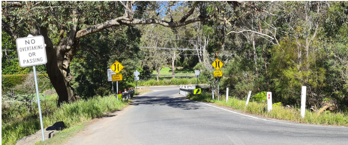
Figure 20 Existing bridge on Morgan Road at Oxford Falls
